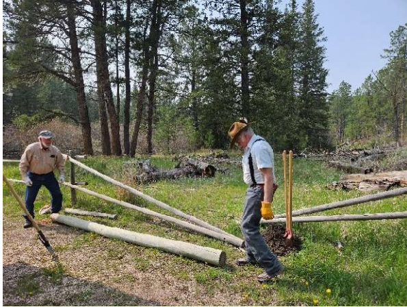
Figures 12 & 13. Ralph and Jim replacing broken post in Iron Creek Horse Camp.
