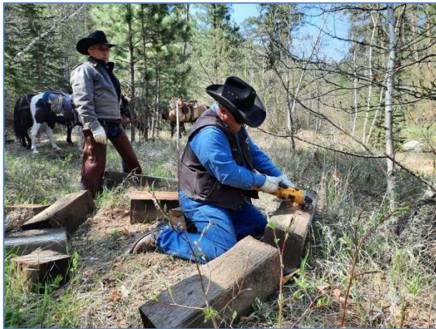
Figure 3 & 4. Doug cutting rebar off of timbers to fit in panniers and loading panniers.
